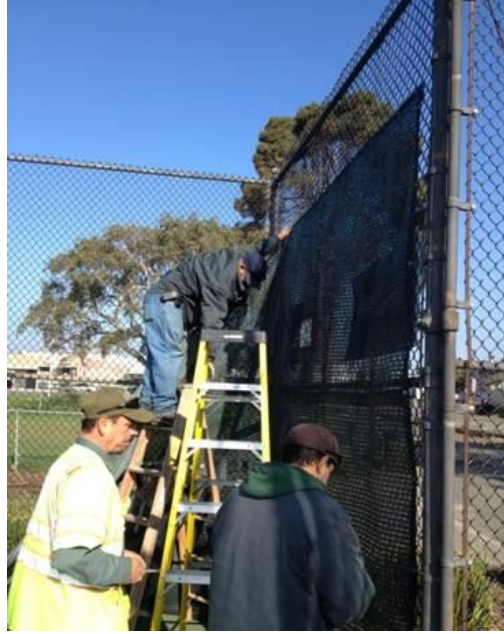
Windscreen Installation at Nicholl Park
