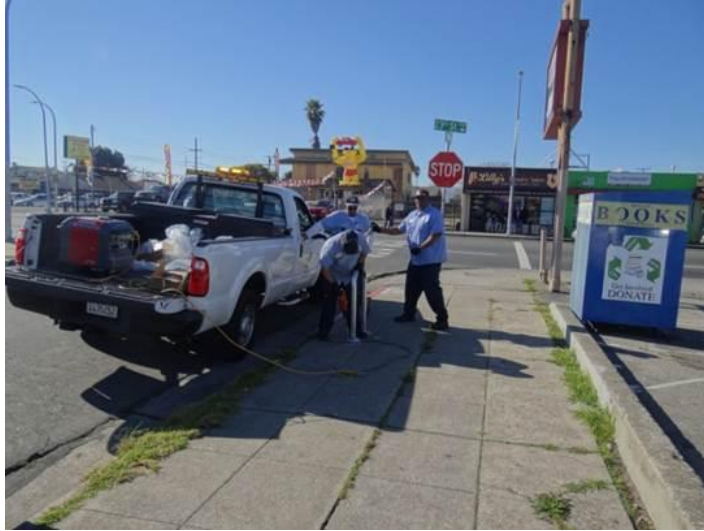
Bicycle Rack Installation
